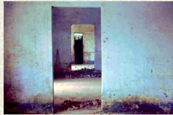
Interior as work begins
